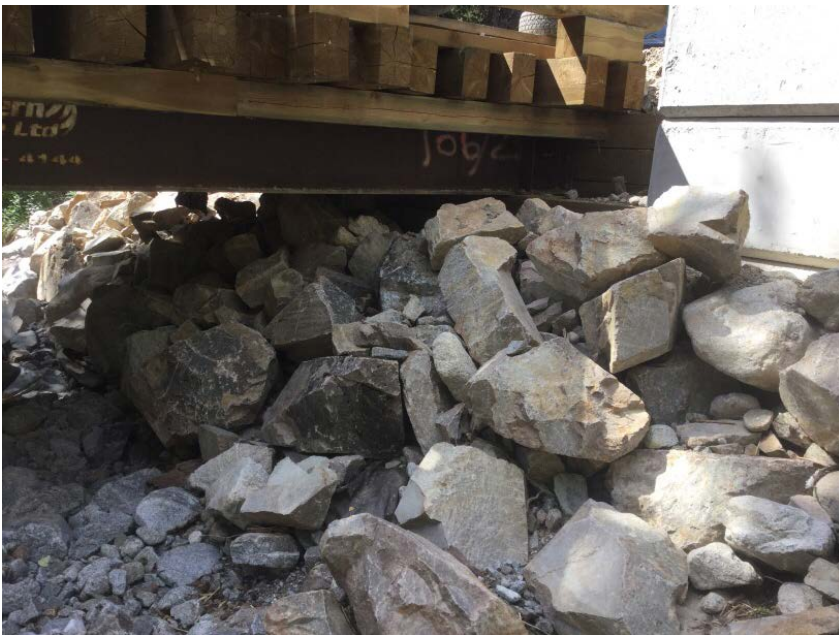
Right Bank Abutment when facing downstream
