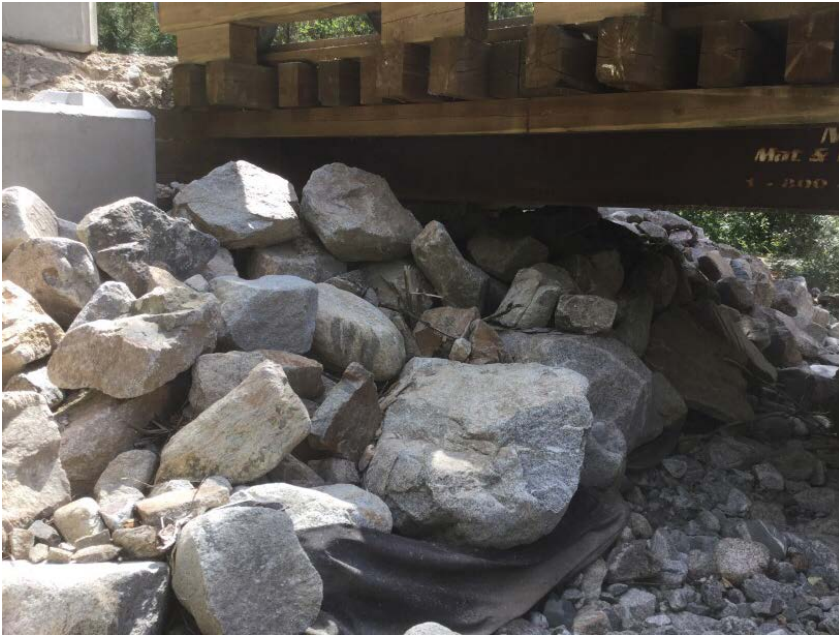
Left Bank Abutment when facing downstream
