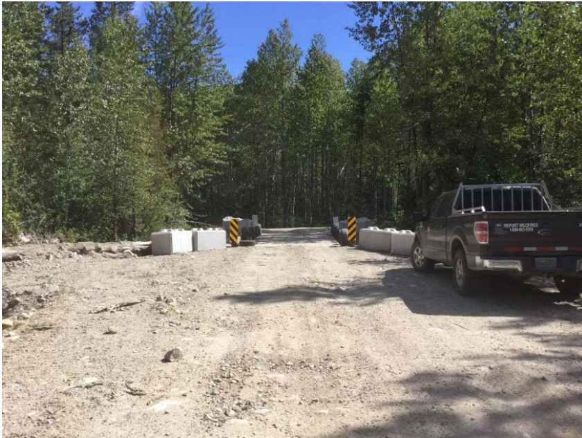
Approach from Right Bank when facing downstream
