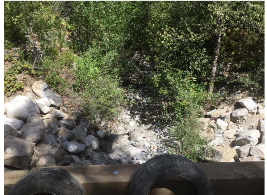
Looking upstream from deck
